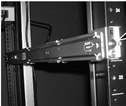
RAIL MOUNTING (FRONT VIEW)
